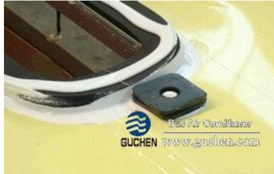
5. Put the shock pads under the condenser.
